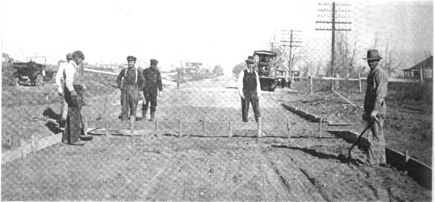
No. 1. Leveling Sub-Grade, Greeley Road.
