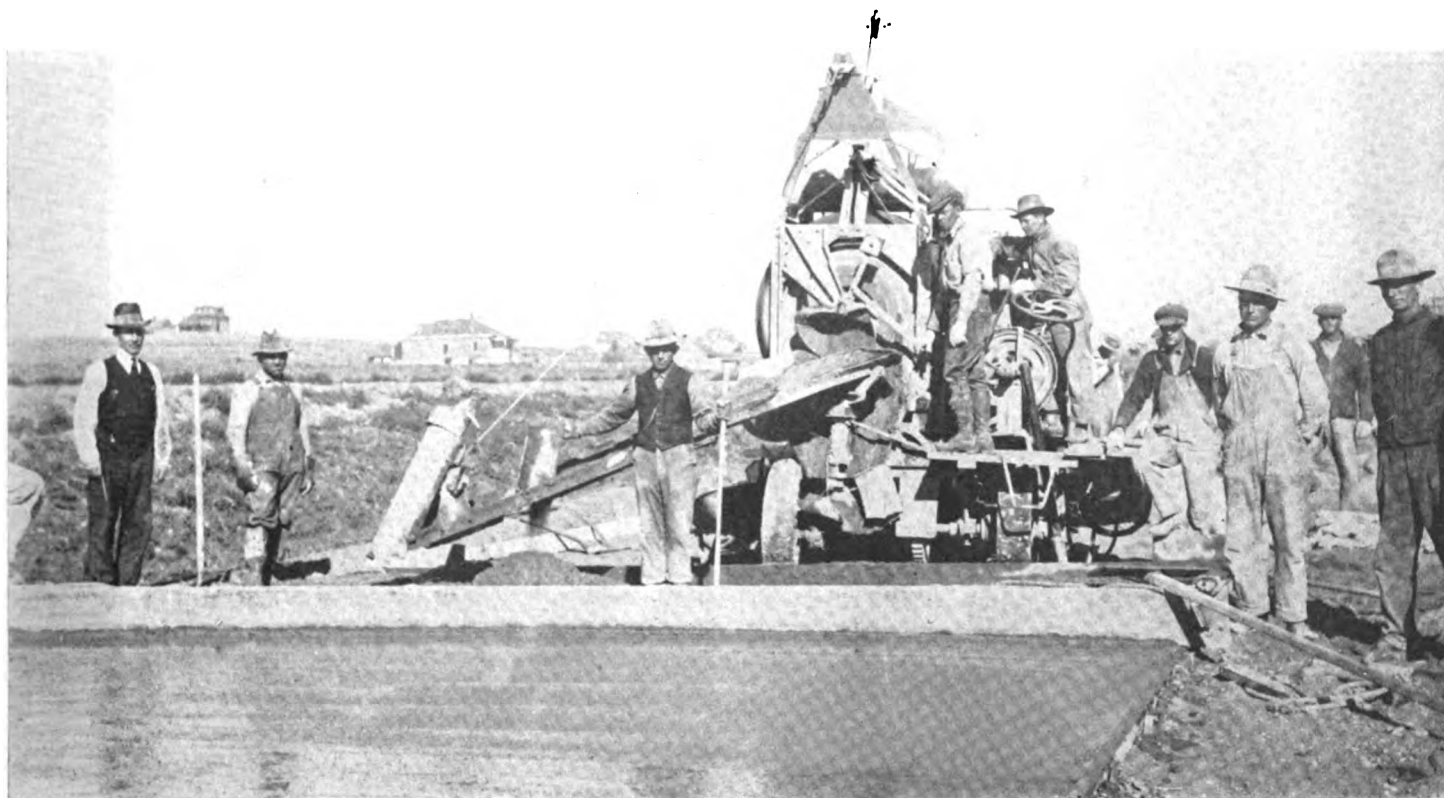
No. 2. Placing the Concrete, Greeley Road.
