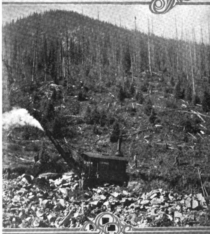
Top Left: Steam drilling outfit on Silverton Road. Top Right: Town of Silverton from Durango-Silverton Road. Below: Powerful steam shovel of caterpillar or tracklayer type at work on this road.
