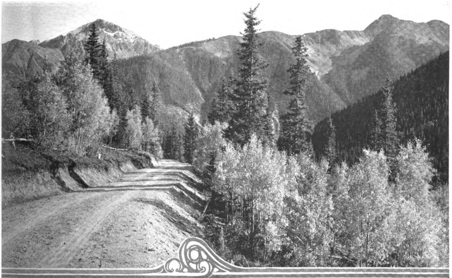
Scene on the Southern Slope of Red Mountain Pass, where the United States Forest Service and the State Highway Department plan the location of nine and one-half miles this season.
