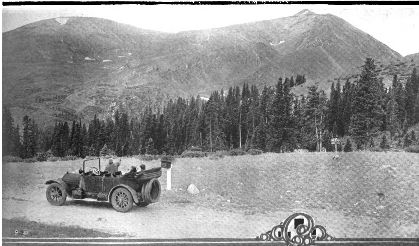
Kenosha Pass. One of the highest and most important passes over the Rockies. Road is being rebuilt here.
