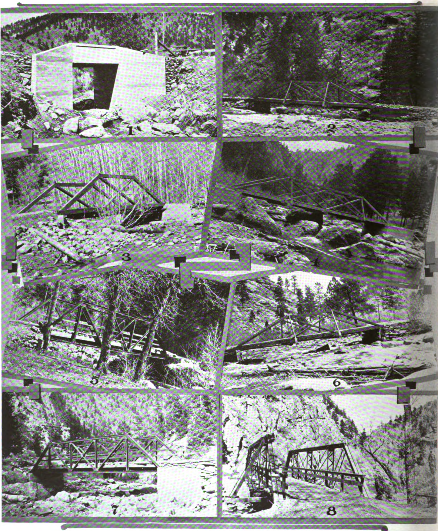
A page of Colorado bridges, showing rugged types of iron and concrete. 1. Bridge at Station 207+00. 2. Bridge at Station 472+50. 3. Bridge at Station 308. 4. Bridge at Station 631+00. 5. Bridge at Station 766. 6. Bridge at Station 664, Colorado F. A. No. 9. 7. Bridge at Station 1060. 8. Bridge at Station 151.
